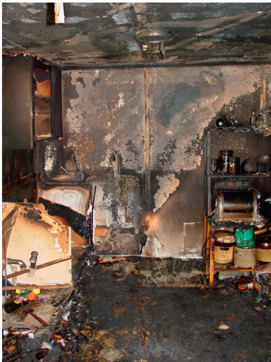
Figure 6 Typical V pattern in a residential fire. The fire originated in a plastic trash can located against the wall in the background. Copyright 2012 from Scientific Protocols for Fire Investigation, 2nd Edition by John J. Lentini. Reproduced by permission of Taylor and Francis Group, LLC, a division of Informa plc.
