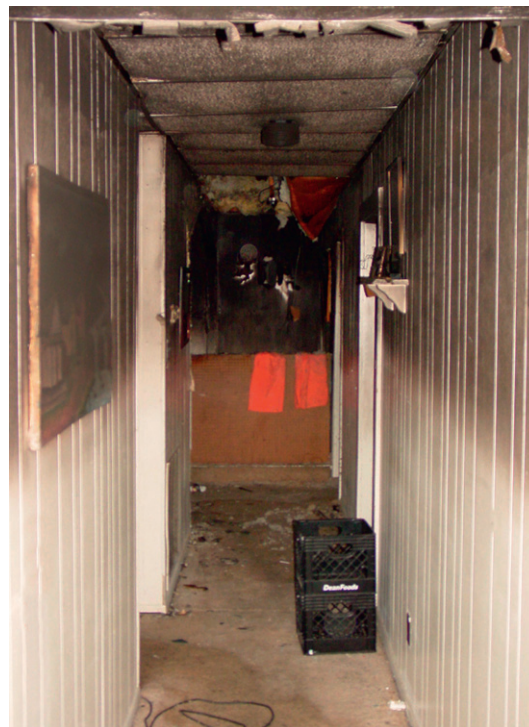
Figure 10 An example of a typical smoke horizon. Photo courtesy of Mick Gardiner, Gardiner Associates, with permission.
