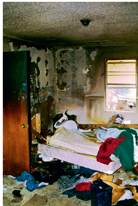
Figure 8 Typical U pattern in a residential fire. The fire originated behind the door at the left side of the photo. Copyright 2012 from Scientific Protocols for Fire Investigation, 2nd Edition by John J. Lentini. Reproduced by permission of Taylor and Francis Group, LLC, a division of Informa plc.
