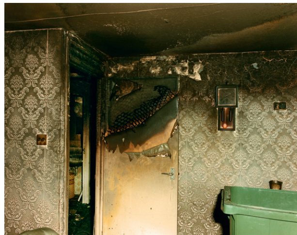
Figure 14 Typical movement pattern through a doorway. Photo courtesy of Mick Gardiner, Gardiner Associates, with permission. Copyright 2012 from Scientific Protocols for Fire Investigation , 2nd Edition by John J. Lentini. Reproduced by permission of Taylor and Francis Group, LLC, a division of Informa plc.
